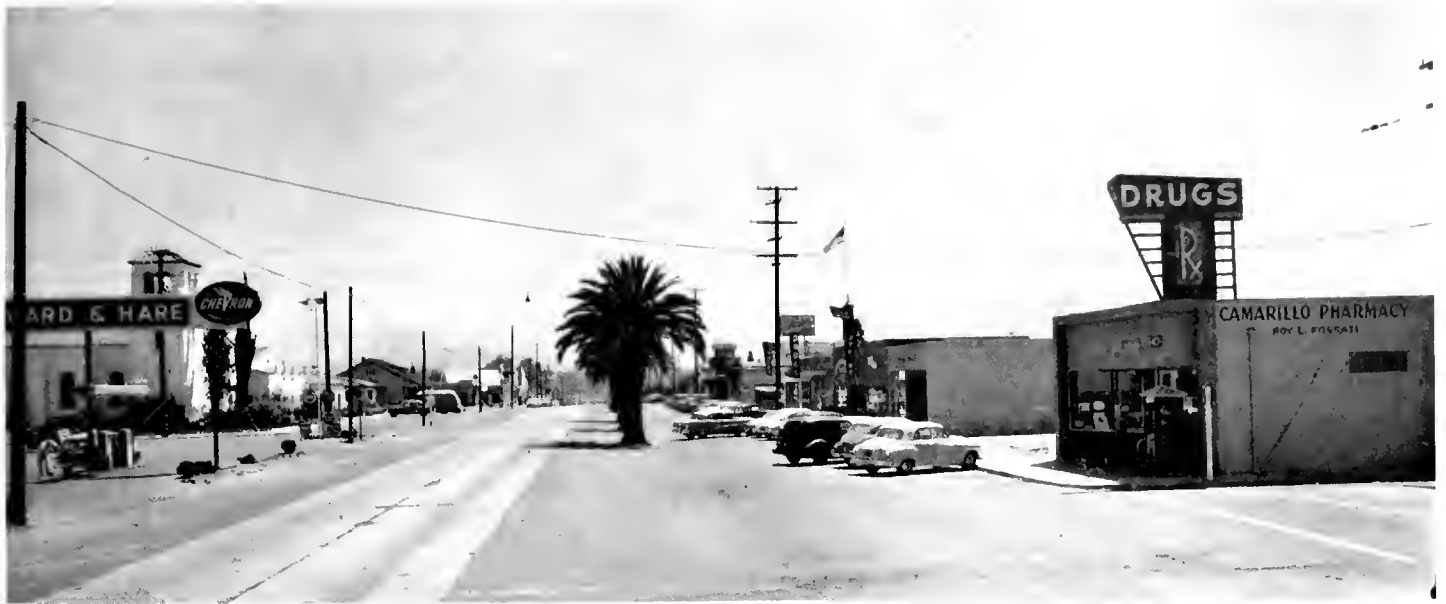
View of business district along old highway route. Many of the commercial structures visible have been built since freeway route adopted.
